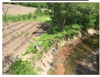
This northeast Kansas creek has migrated through the edge of its riparian forest. The landowner recognized that without the protection of tree roots, bank erosion was about to become a problem. He ensured short-term bank stability by anchoring large dead trees and live willow cuttings along toe of the bank. Long-term bank stability will be maintained here by the several rows of hardwood trees he planted along the edge of the field.
