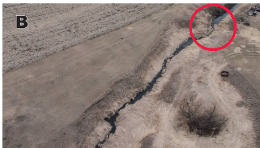
Stage 4. Channel appears to be widening after incision
