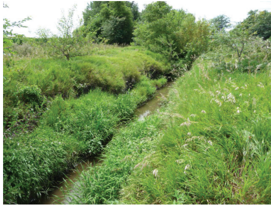
Figure 16. Active bank slumping along left banks.
