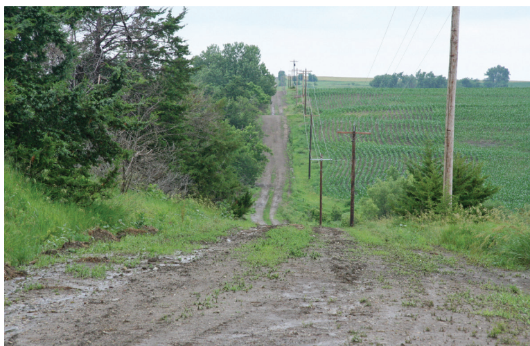
Photo 5. Unimproved roads were prevalent in all three watersheds and may be significant sources of sediment.
